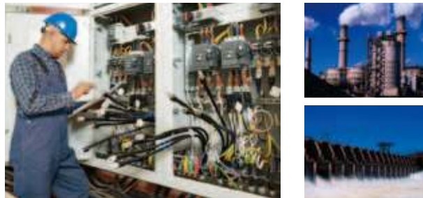
Supports high voltage systems around the world
